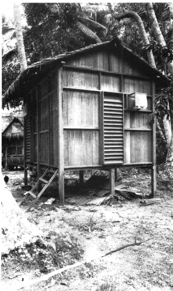
Fig. 1. Experimental hut in Jalan Baru, Penang.
